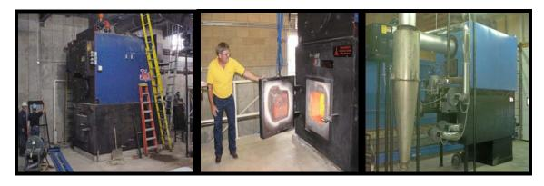
Figure 7 – Boiler, Combustor and Multi-Cyclone<sup>58</sup>
